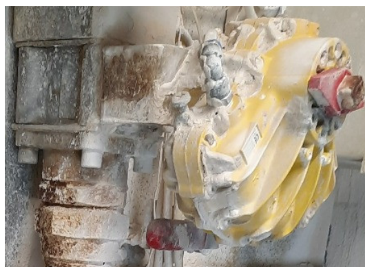
Kinetrol actuator on valve installed on highly abrasive kaolin slurry feed pipes.
